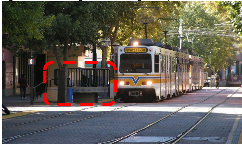
Figure 28: SacRT Light Rail Mini-High Ramp
